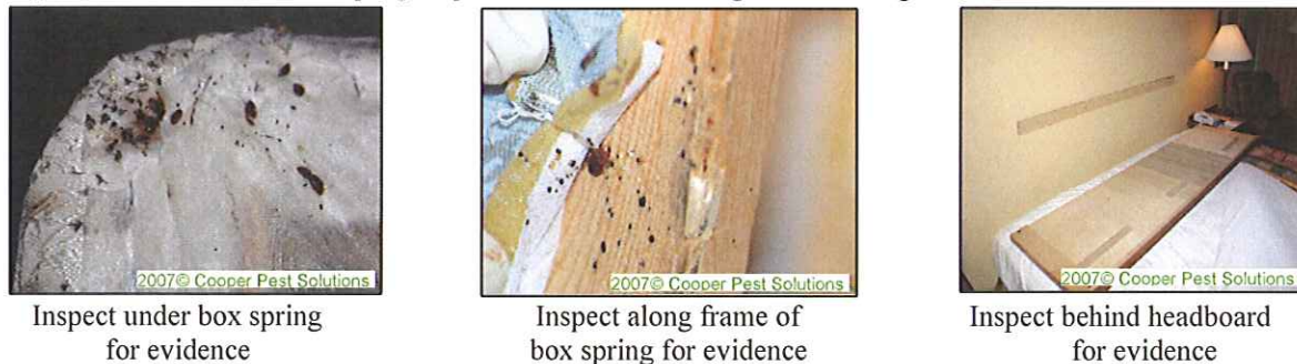
Figure #2 Routine housekeeping inspections for obvious signs of bed bugs
