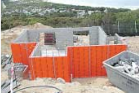
Photo 1 Kordon TB - full retaining wall
