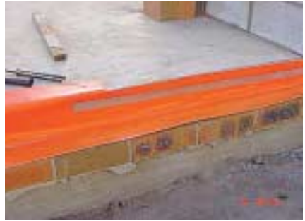
if tiling is to extend to slab edge Kordon TB is installed as shown - secured with gal hoop-iron/strapping.
