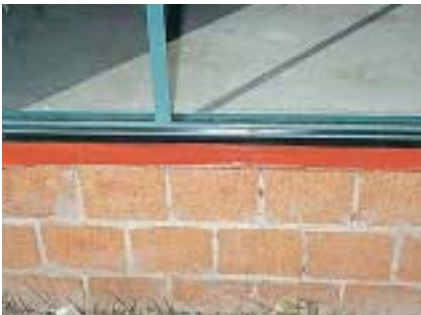
renderlok secured to masonry with approved concrete nails. - (15mm length preferred)
