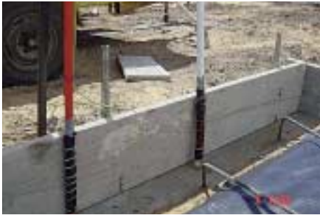
photo 1 before the slab pour showing black plastic facing out large overlaps
