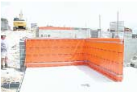
Photo 3 Kordon TB - internal wall treated
