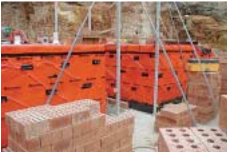
Photo 2 Kordon TB - retaining/stepdown
