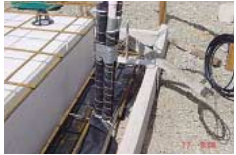
photo 2 showing multiple pipes each protected with Kordon
