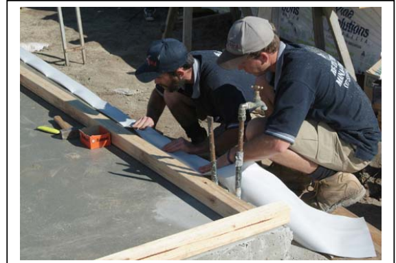
HomeGuard DPC 0.5mm product being installed in the perimeter cavity
