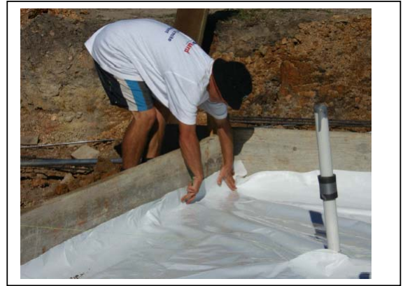
HomeGuard TMB 0.2mm sheet product being installed
