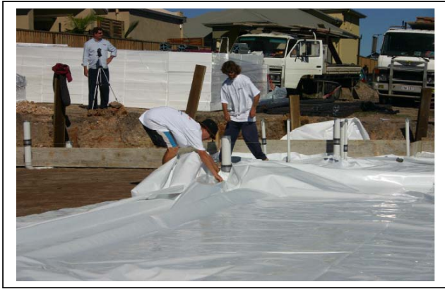
HomeGuard TMB 0.2mm sheet product being installed
