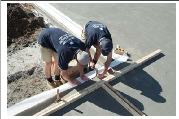
HomeGuard DPC 0.5mm product being installed in the perimeter cavity
