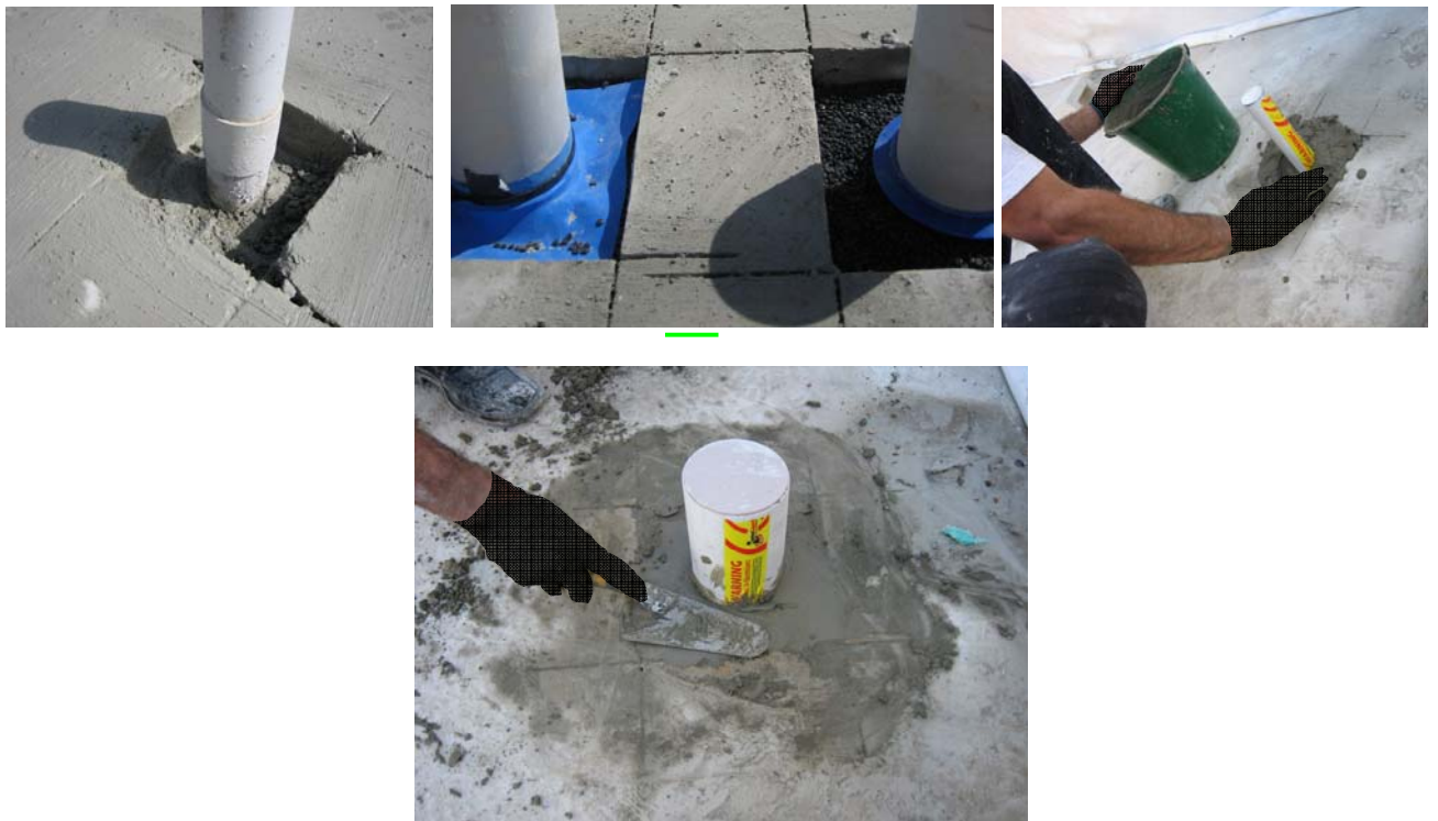
Above and Left : Using GT for retro protection of service pipes.
