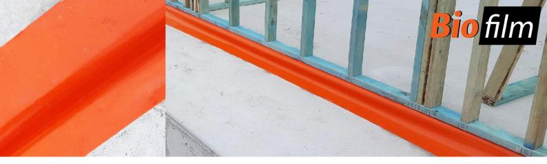
Biofilm is an Australian owned and manufactured flexible sheet material designed to be used as a component of a Termite Management System to deter concealed entry of subterranean termites from the soil into a building.
